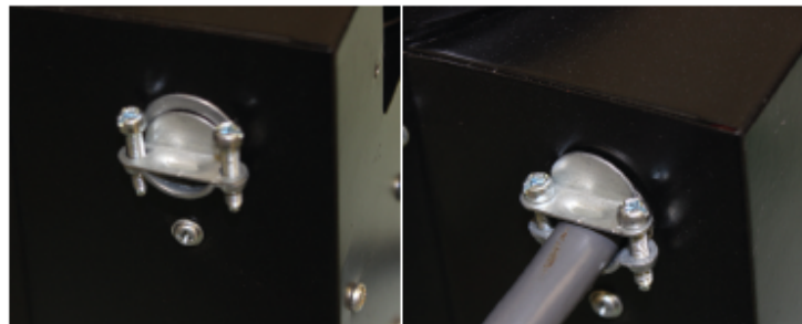
Figure 9: Installing cable fitting to heater
