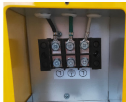
Figure 10 Removing wiring cover exposes wires When wiring with 2 conductor cable with ground, the white wire must be marked black.
